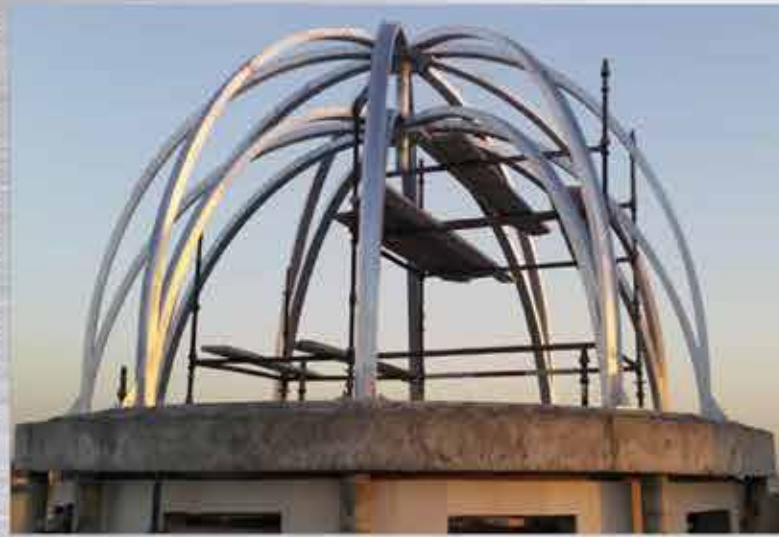
STEEL DOME, AL SHIBANI VILLA, MUHAISNAH- ADNAN SAFFARINI CONSULTANT
