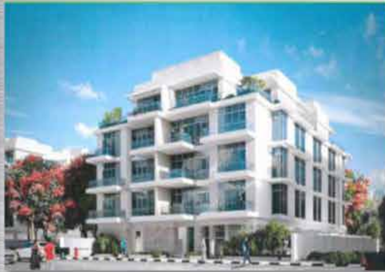
ROOF STRUCTURE G+4 # 29 BUILDINGS POLO RESIDENCE - NAD AL SHIBA
