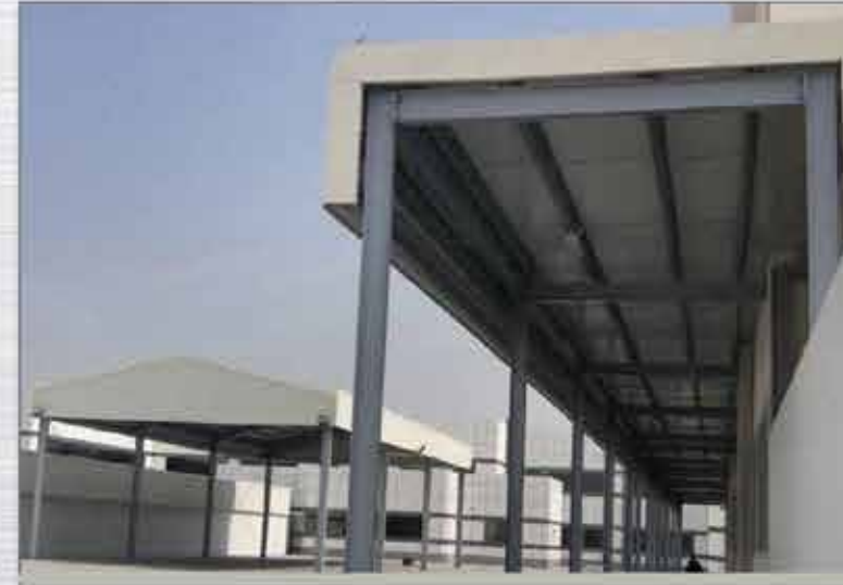
ZUHOOR SCHOOL WALKWAY, SHARJAH - ADNAN SAFFARINI CONSULTANT
