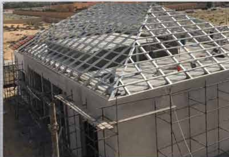
ROOF CANOPY, KHAWANEJ-ADNAN SAFFARINI CONSULTANT
