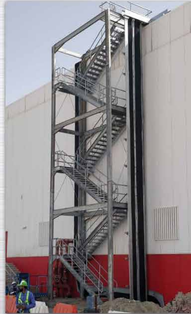
STAIRCASE, ARAMEX LOGISTIC DUBAI SOUTH
