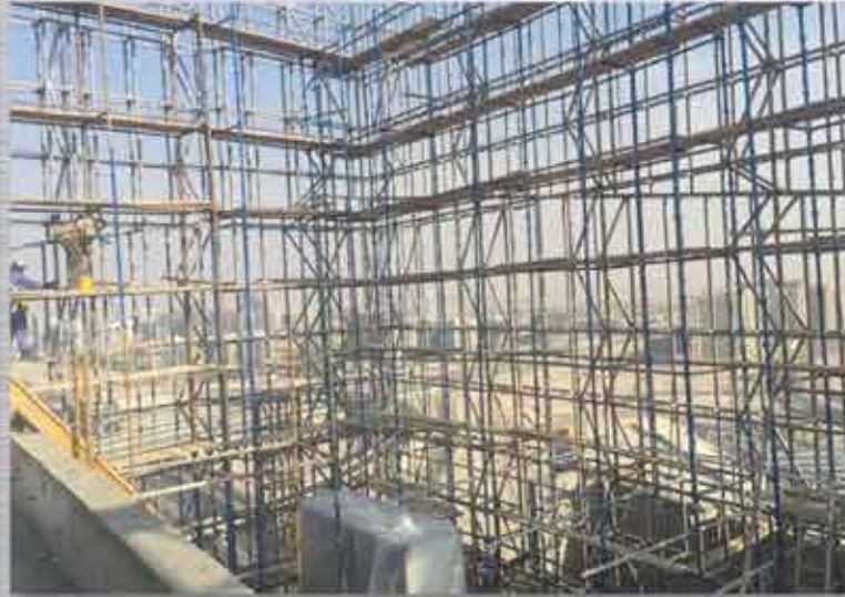
TIGER GENERAL CONTRACTING - STEEL CANOPY G+29- JVC LACASA CONSULTANCY
