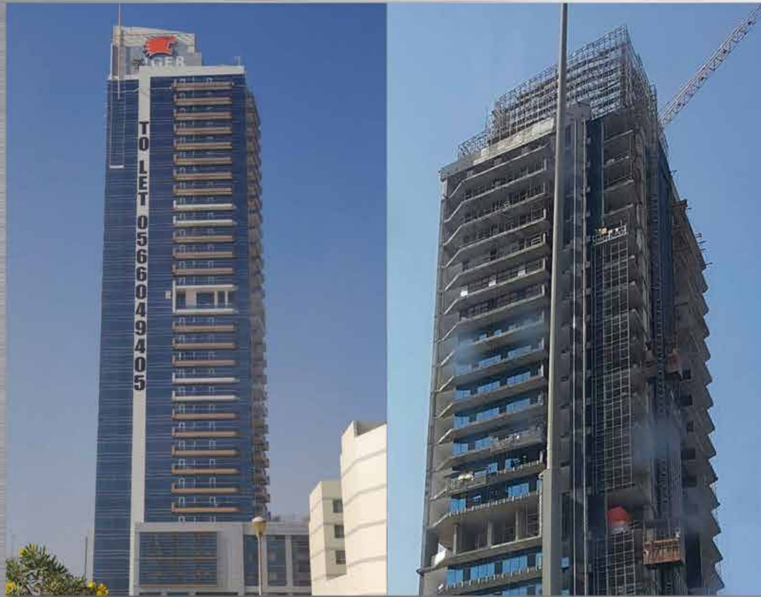
TIGER GENERAL CONTRACTING STEEL CANOPY G+29- JVC LACASA CONSULTANCY
