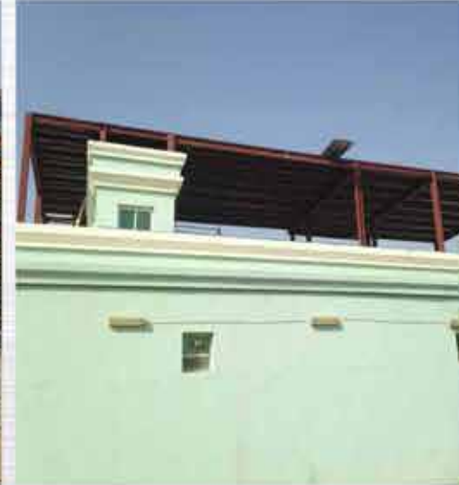
STEEL STRUCTURE FOR ADDITIONAL FLOOR
