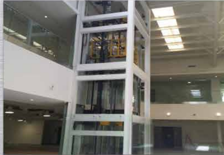
ELEVATOR, MALL OF THE WORLD JUMEIRAH- LACASA CONSULTANCY
