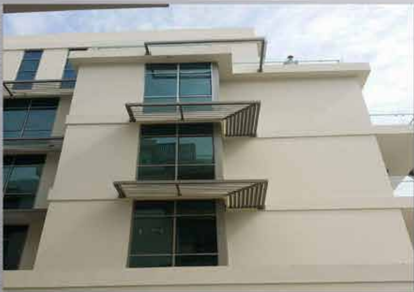
HOT DIP GALVANIZED WINDOW SHADING FRAME LOCATION: POLO RESIDENCE 29 BUILDINGS AT MEDAN, DUBAI UAE CONSULTANT: ARCHCORP ARCHITECTURAL ENGINEER MAIN CONTRACTOR: TECHNICAL ARCHITECT CONTRACTING LLC
