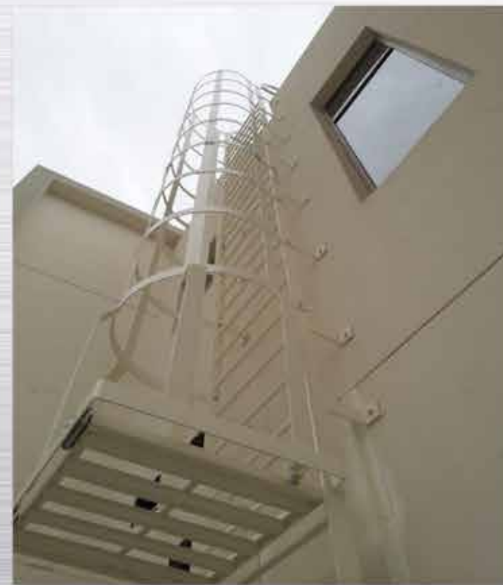
CAT LADDER WITH SAFETY CAGE AND DOOR G+1 - 47 VILLAS & 34 TOWN HOUSES AT AL FURJAN DUBAI UAE CONSULTANT: ARKIPLAN CONSULTING, ARCHITECTURAL & ENGINEERS MAIN CONTRACTOR: TECHNICAL ARCHITECT CONTRACTING LLC
