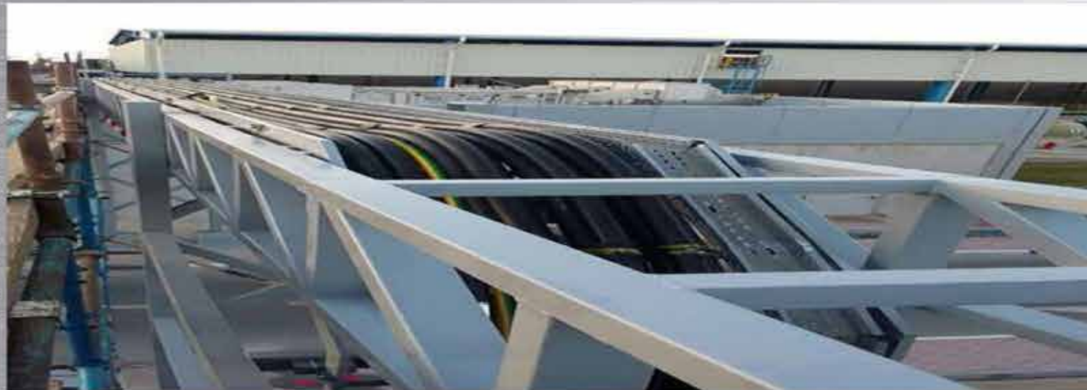
DEWA M-STATION SOLAR POWER PROJECT
